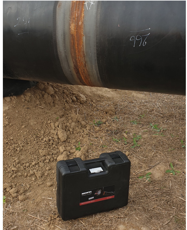
Figure 4. Training on the job before coating. MONTI's toolbox is ready for use.
